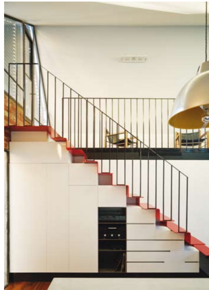
A folded steel plate stair wraps over cabinetry to make the study accessible.
